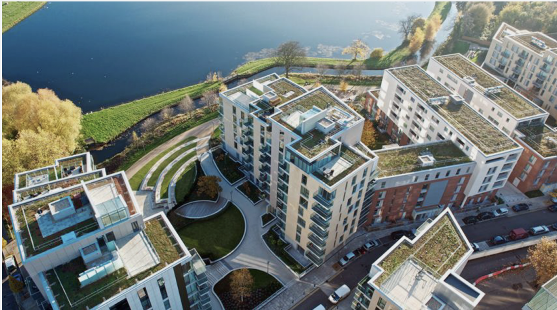
Woodberry Down's green roofs.
